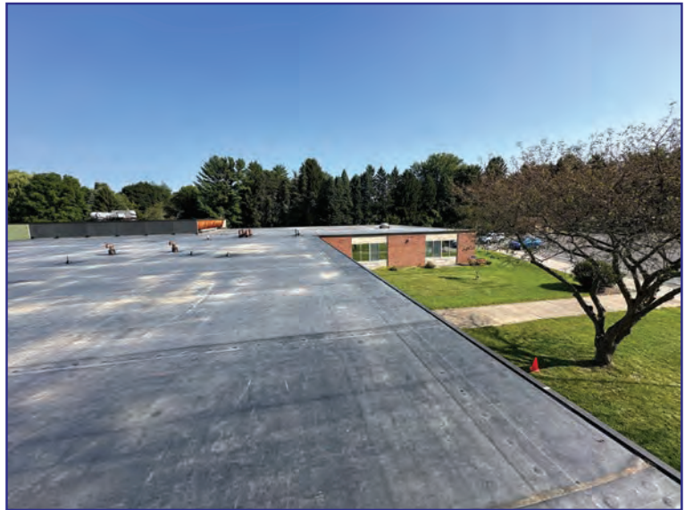
A view of the completed new roof
